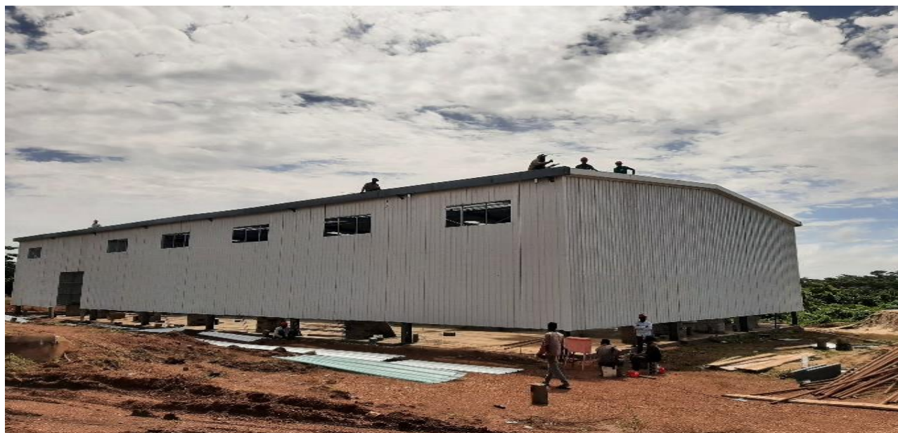
Figure 1: Feed mill component of the poultry factory nears completion
